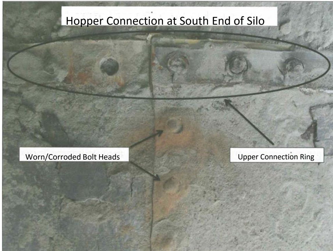
Photo showing interior of "Sand Plant Fines" Silo
