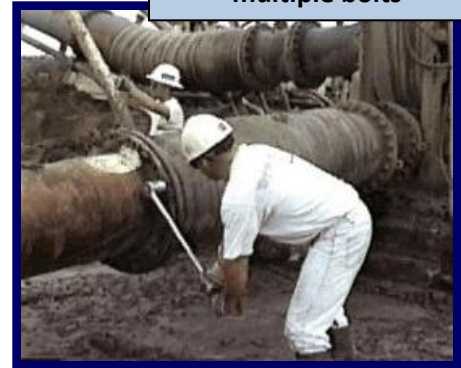
Removing /tightening multiple bolts
