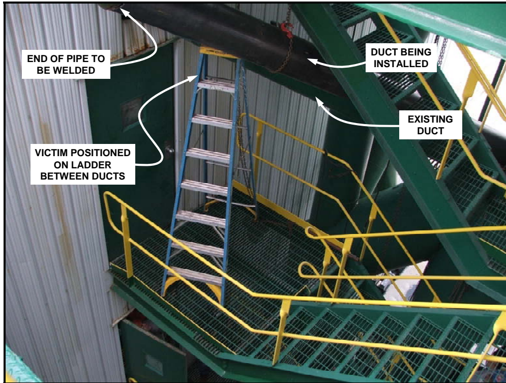
Figure 1 – Work area location
